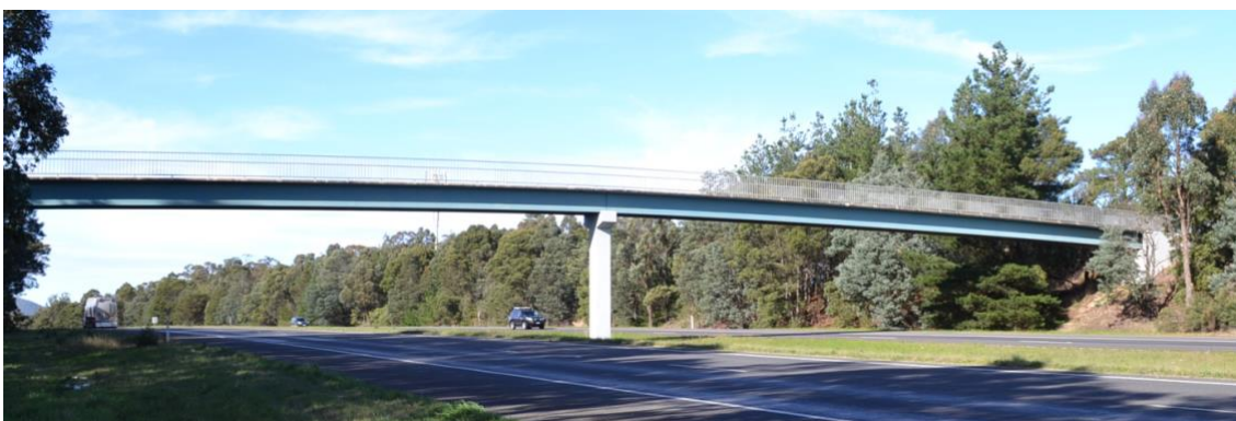
Nerrina Foot bridge
