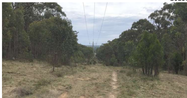
Cleared area under the power lines and the water easement. Image 18 th December 2023
