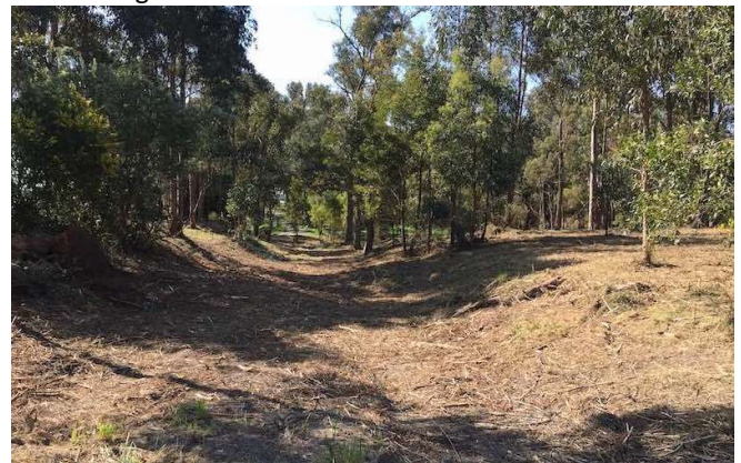
The Ballarat to Buninyong Railway cutting looking north from Horwood Avenue. Image: 28 th September 2023.
