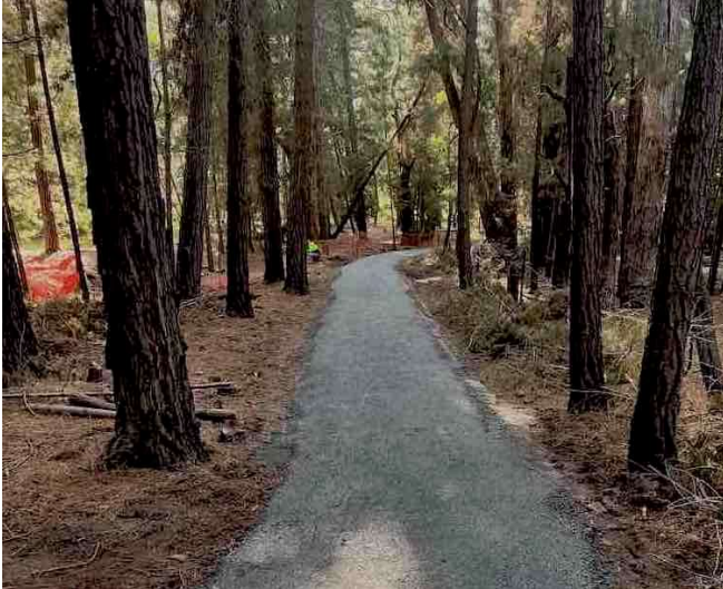
Newly topped Bunny Trail. Image: Courtesy of Crackers, 22 nd May 2023.
