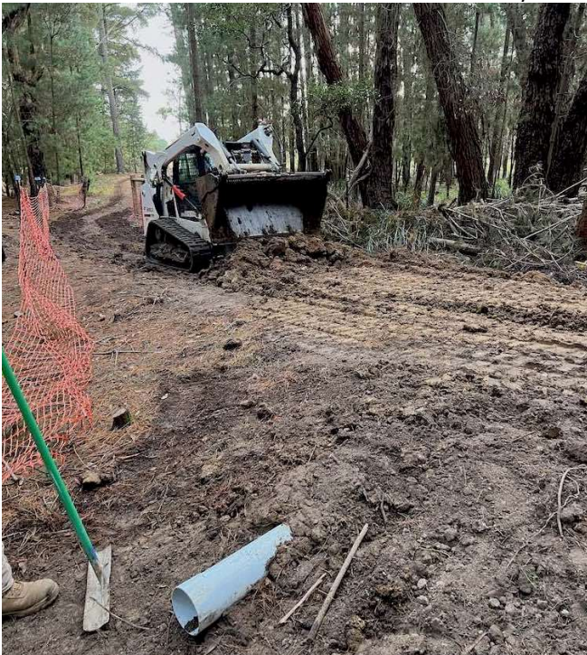
Drainage pipe and fill construction. Image: Courtesy of Crackers, 22 nd May 2023.
