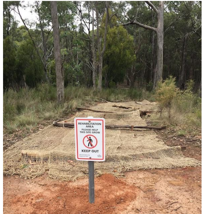
Restoration ground works on top of Red Hill. Local tree and ground cover seed was collected within the Park and spread under the installed matting to promote regrowth.
