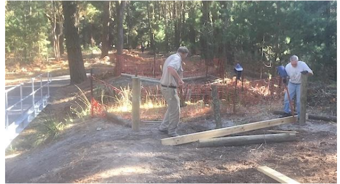
Bob and Bernie installing the safety rails. Image: April 4 th 2023
