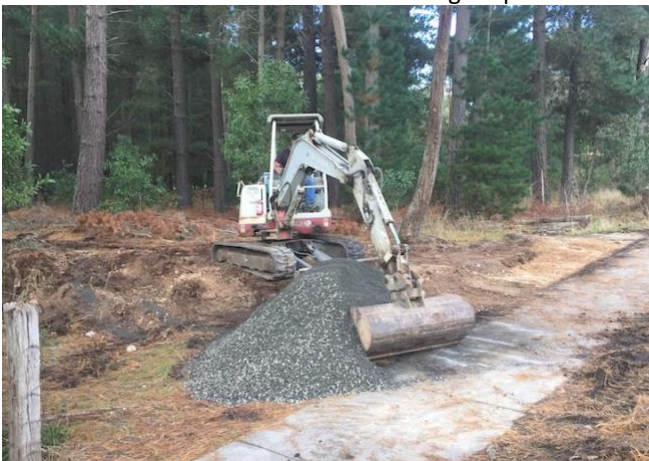
Earthworks at the trail entrance. Image: April 18 th 2023
