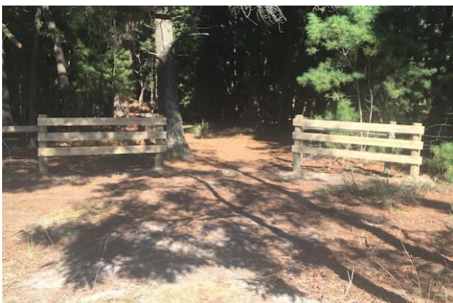
Parks Victoria's new North entrance to the "Bunny Trail" at the Recreation Rd Bushland Reserve. Image: April 24 th 2023
