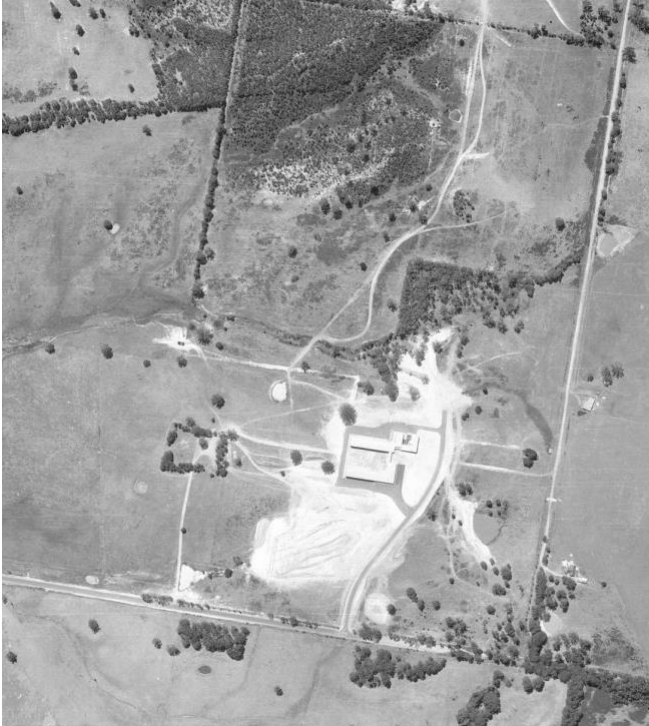
First buildings in a very bare landscape at Mt Helen. Image: 1970
