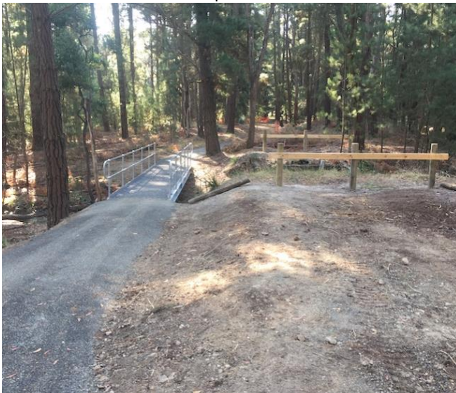
The installed bridge and safety rails. Image: April 4 th 2023.
