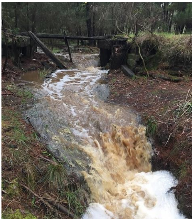
Toms Creek under the rail bridge at 55 Recreation Rd. Image 7 th October 2022
