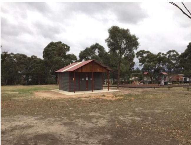
The new toilet block at Sparrow Ground Spencer St Canadian. May 2022
