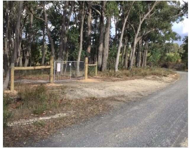
Installed gate on Katy Ryans Rd. Image April 7th 2022
