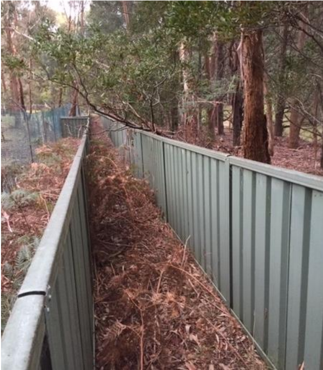
3) The Koala passage link on the westside of the Eastbound Lanes of the dual lane Ballarat highway turn off. Image 25 July 2021
