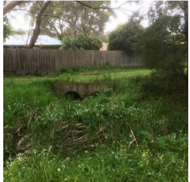
Image 47: The partly blocked outlet into Canadian Ck. In this increased heavy rain fall era, what flow rates was this 40 year old piping was designed for? October 2019.
