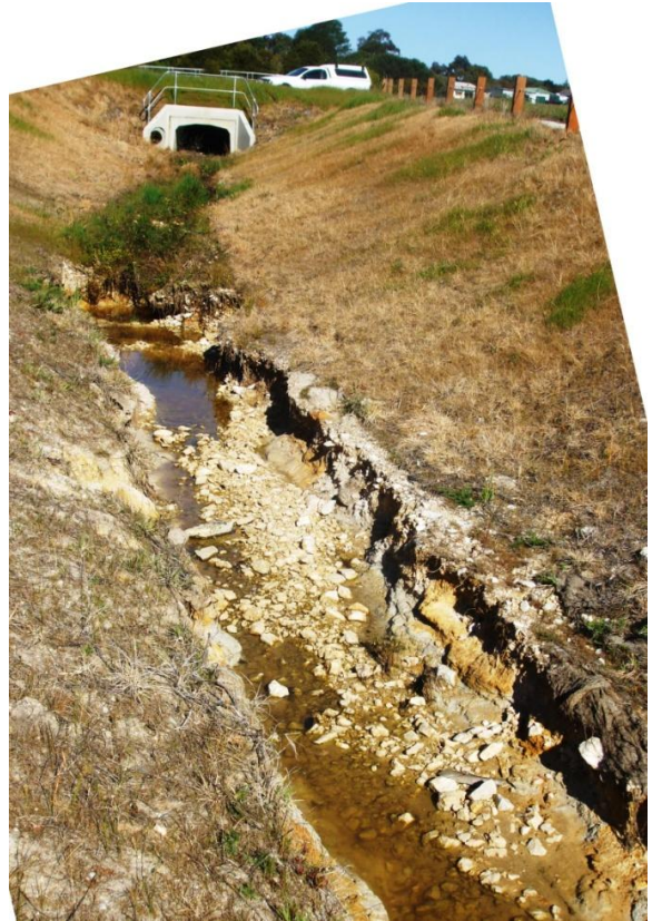
Image 21: Looking east at erosion in recently constructed creek (drain)
