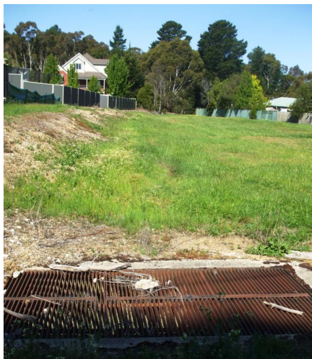
Image 45: Piped section of Unnamed Creek 3 below the railway bridge. Note overflow grating and provision for overland flow. October 2019.
