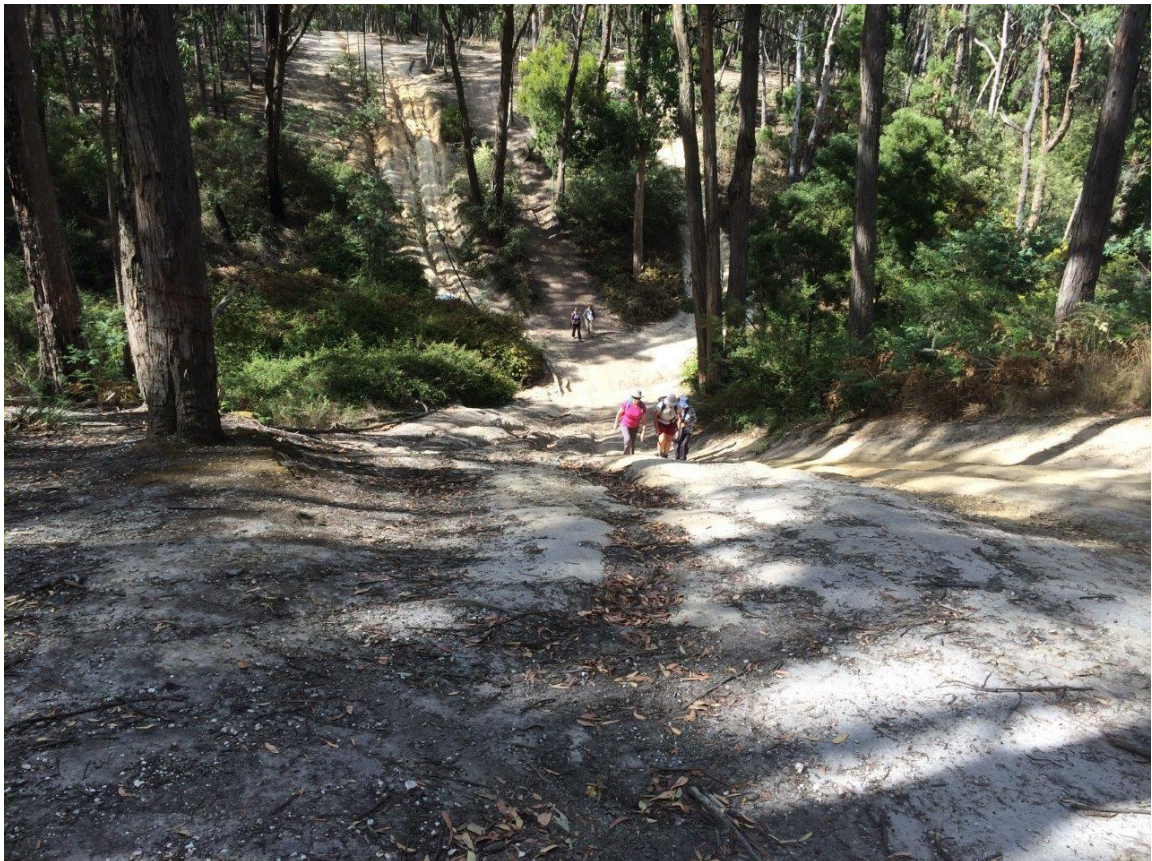
Image 50: The Central Highlands Water easement across Unnamed Forest Creek. The access track has been badly damaged by 4WDs and was scheduled for restoration in winter 2019. J Petheran 2014.
