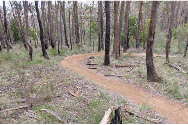
Repaired trail. Images 1 st December 2021
