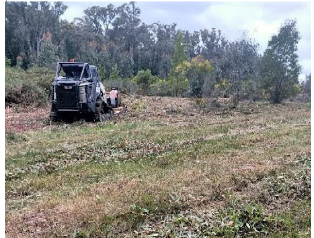
Eco Blade at work on 25 th October 2021. Image courtesy of Rex.
