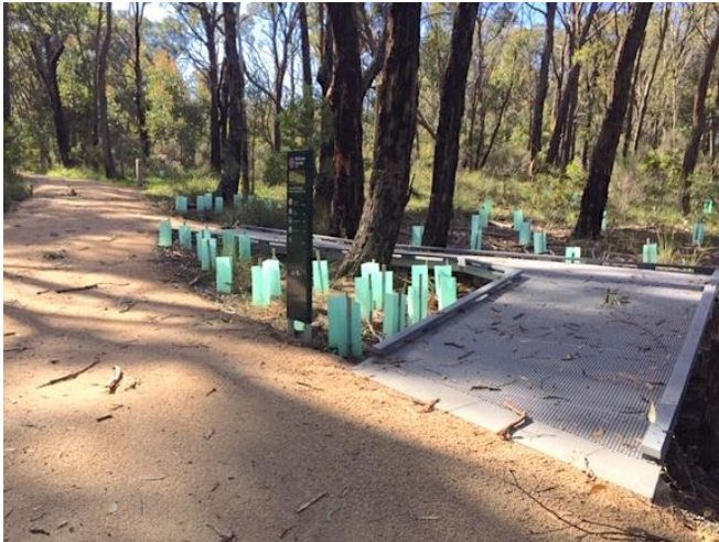
The wheelchair friendly walkways and granite sand topped path on the trail. Image 30 th October 2021.
