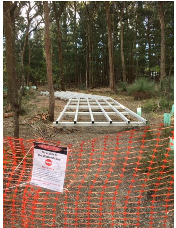
Boardwalk construction in the wetland loop. Image August 29 th 2021
