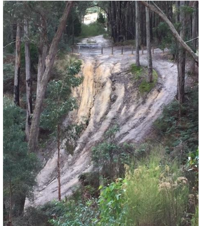
Damage on the Gorge north face with the newly installed gates and fence in the background. Image 26 th May 2021.
