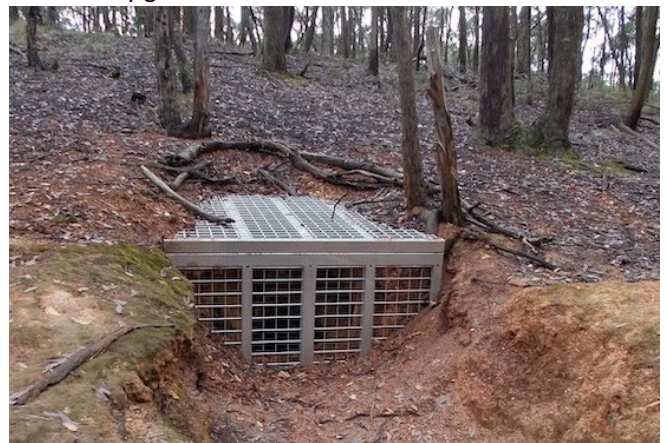
Adit safety grill Image 25 th March 2021
