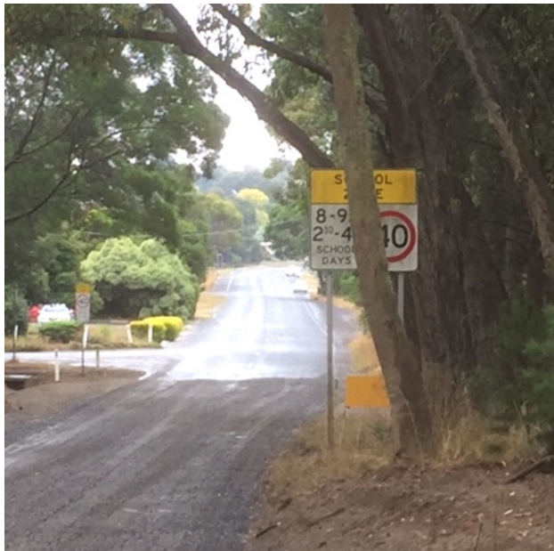
The obscured 40kph zone sign on the east end of the school zone. Image 8 th March 2021
