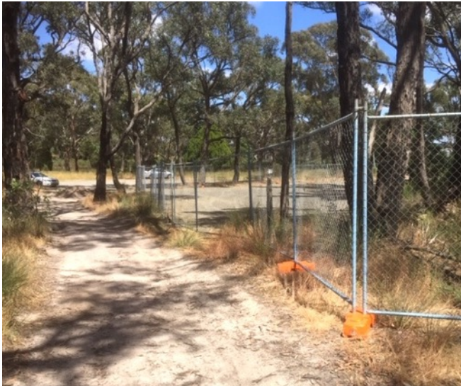
Image: Fencing around Car Park area construction zone. 20 th December 2020.
