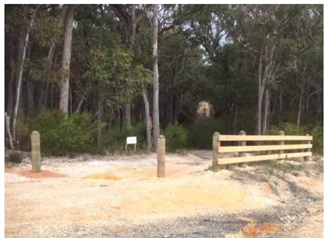
Works on the Olympic Avenue. Image 27 th April 2021
