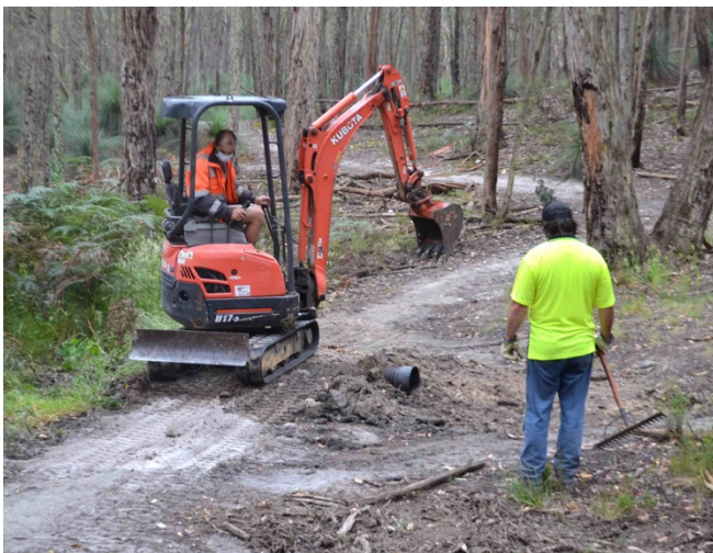
First day drainage works near Conglomerate Hill. Sunday November 22 nd 2020
