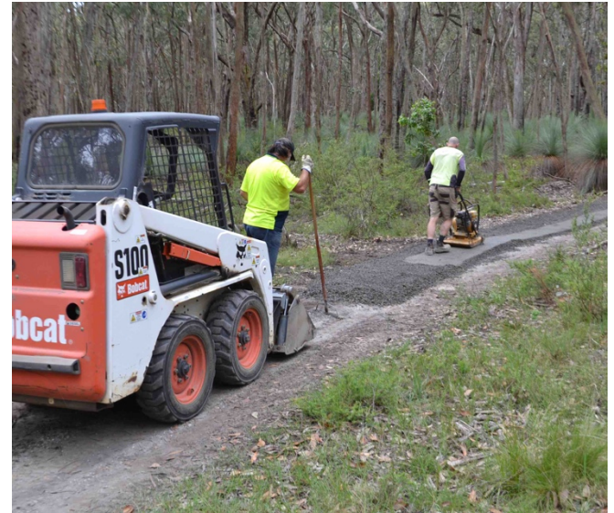
Third day. Spreading and compacting the track surface.
