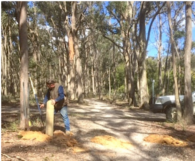
Bollards being installed 3 rd September 2020
