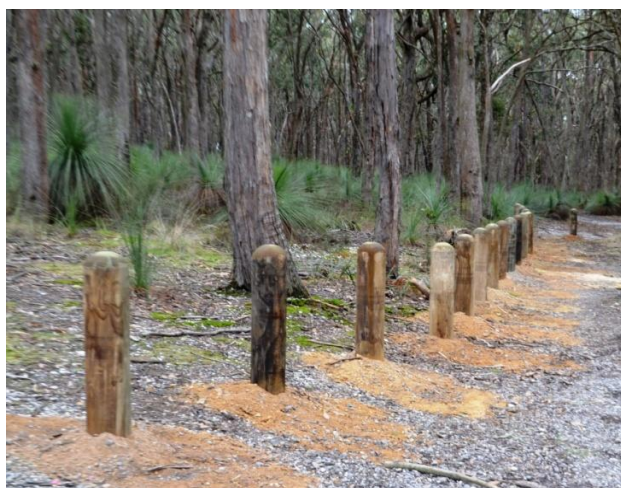
Bollards placed to restrict access.
